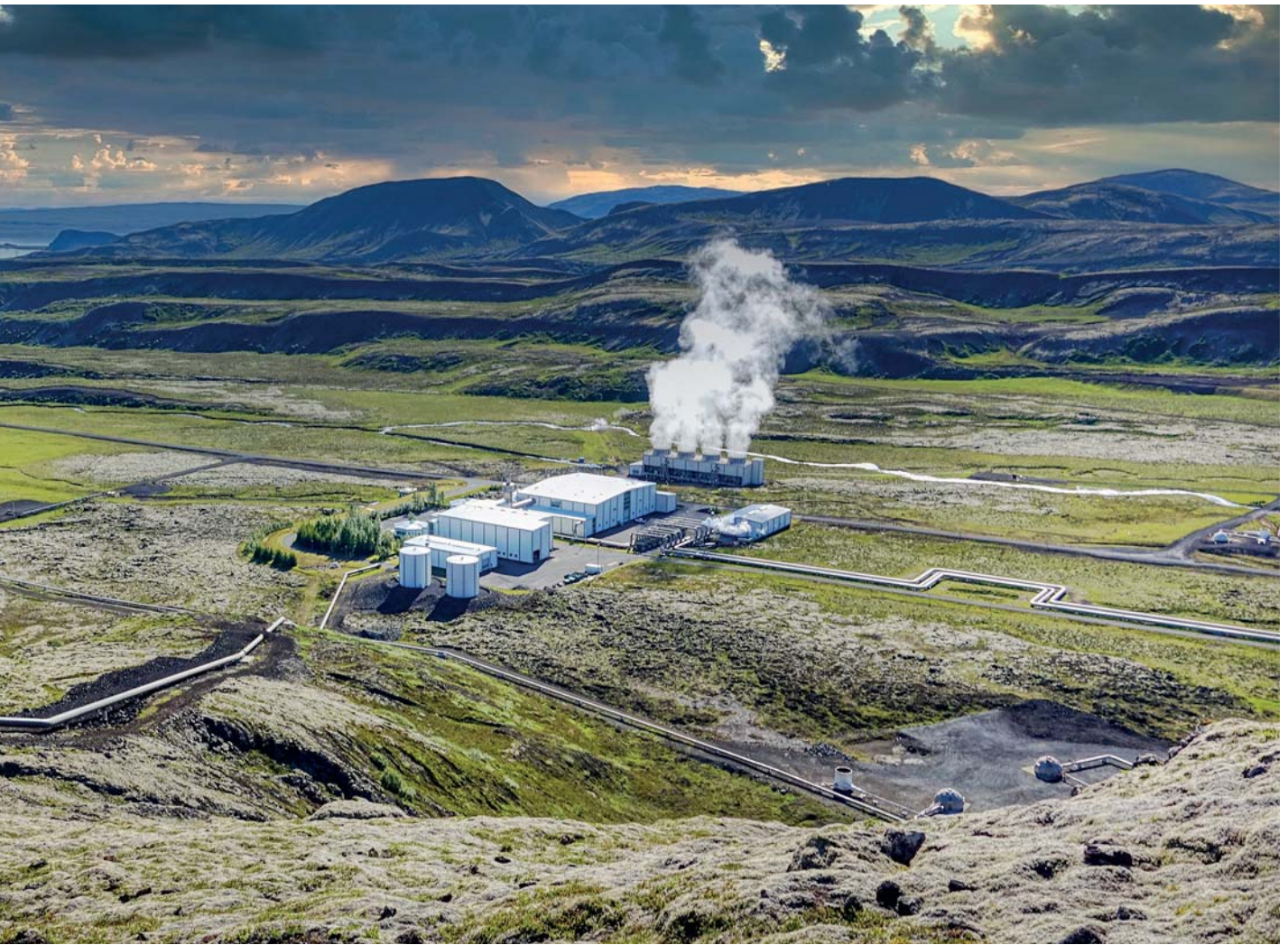
A geothermal power station in Nesjavellir, southern Iceland, which has reduced consumer energy bills amid cost-of-living pressures
